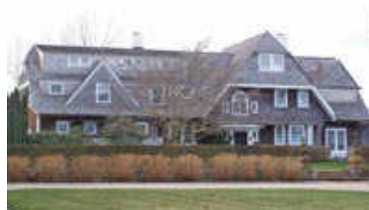
High Wicket (Sowanniu, Chuckle Hill, Greyside North) , 1900
