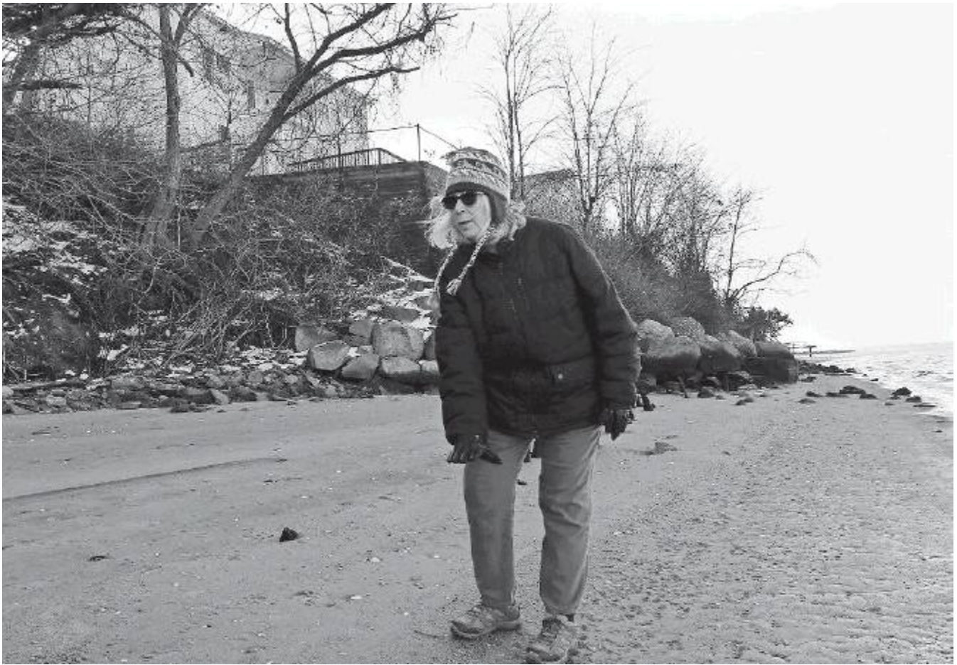
Janet Freedman of the Rhode Island Coastal Resources Management Council on a beach that has been eroding near Rose Larisa Park in East Providence. The area will be used to test a new erosion-abatement system. [THE PROVIDENCE JOURNAL / BOB BREIDENBACH]
