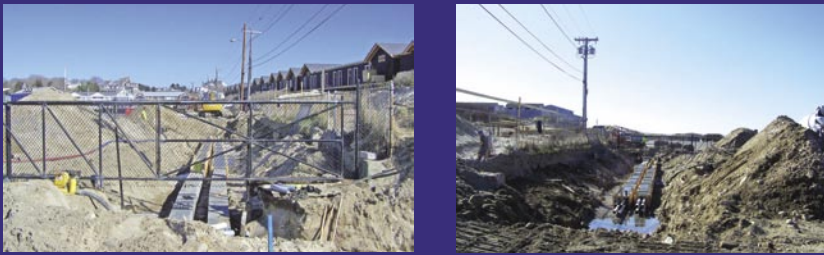
April: Underground Duct Bank Construction, Phase 1A
