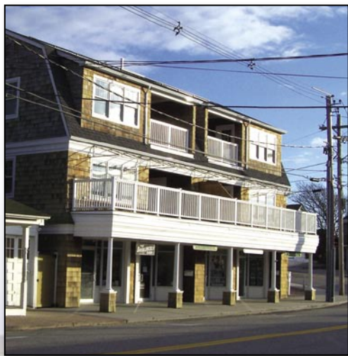
124 Bay Street, Watch Hill. The building's "break-away" first floor walls are indistinguishable from the street. Photo Richard C. Youngken
